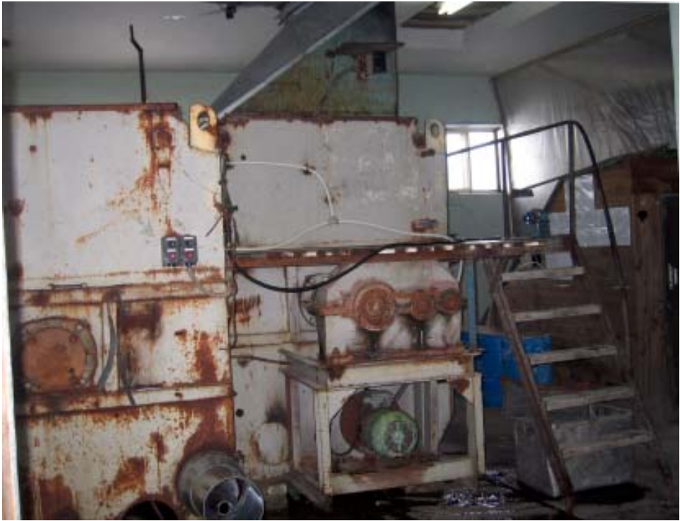
Fig. 13. The ends of two single shafted mixing machines used to pasteurize, cool, spawn and fill plastic “giant sausage” growing containers. (Russia)
