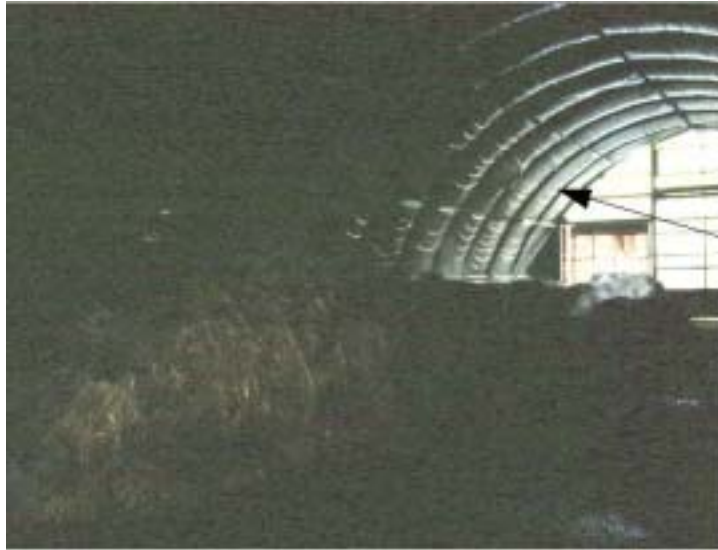
Fig. 3. Building with insulation covered by a plastic vapor barrier.
