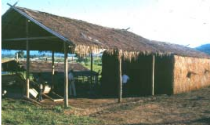
Fig. 4. Growing buildings constructed of bamboo, polyethylene sheet and straw.
